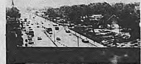
Building demolished; southbound lanes established, balance of former buildings now empty areas. St. Ignatius and Trinity Lutheran Churches visible.
