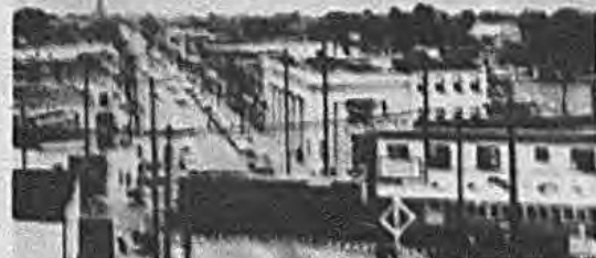
1958 - Broadway - 107 - Before railroad trestle and road widening by demolishing the west side of street. Photo by F. Mallet
