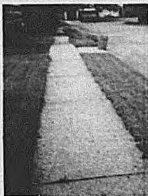
Many sidewalks are in a deplorable condition.
