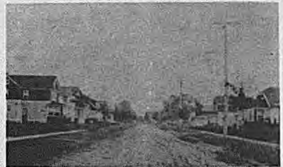
Harding Ave. - 1924, from #43 looking south toward Plainview Rd. - on muddy days movers were stuck hubcap deep.
