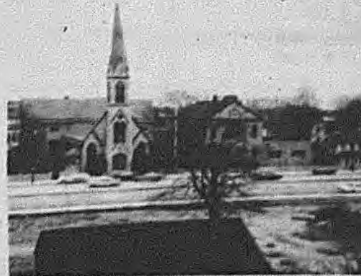
1968, St. Ignatius Church and Old School House, Now Parking area. Photo was taken from Nicholas School Attic east window two days before school demolition.
