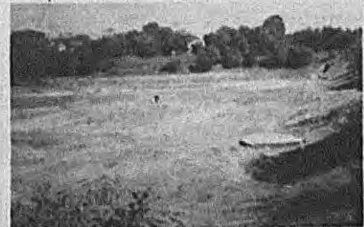
A beautiful sight for sanitary engineers - water supply pros, is the cleaned recharged water basin (sump) east of LILCO's headquarters. White sand expanse free of four feet of 40-year sludge, will return storm run-off water to the water-table, eventually.
