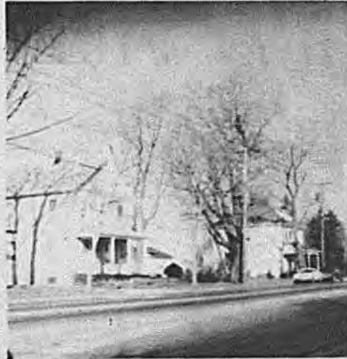
1978 Woodbury Road Houses as seen above, but not visible from former Fountain area today. Photo by Bill Clark
