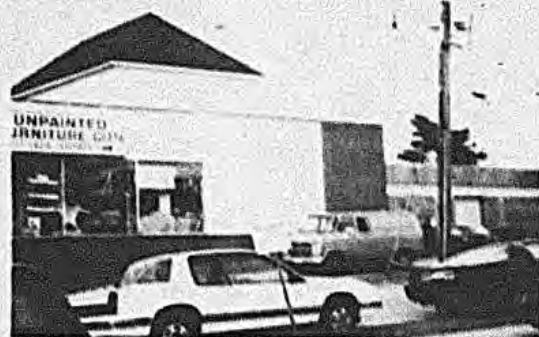
Present day photo - Dome of building and garage area in back - Lenox Ave.
