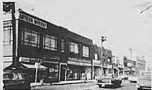
Entire new building after fire with Bahrenburg Bakery on corner later Engler's
