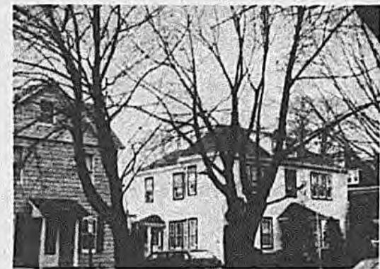
Lower Photo Same 2 homes moved now on E. John St. Photo by Bill Clark
