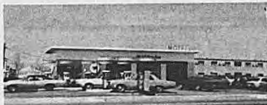
Lower photo: Same area - Old Country Road after widening. Wantagh Parkway to the left.
