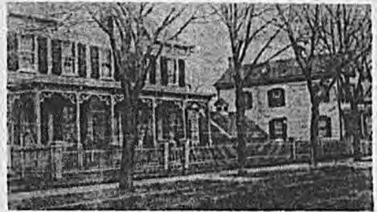
Braun House with Ice House between the houses. Next to house on left later would be Bohack Grocery and Socony Gas Station
