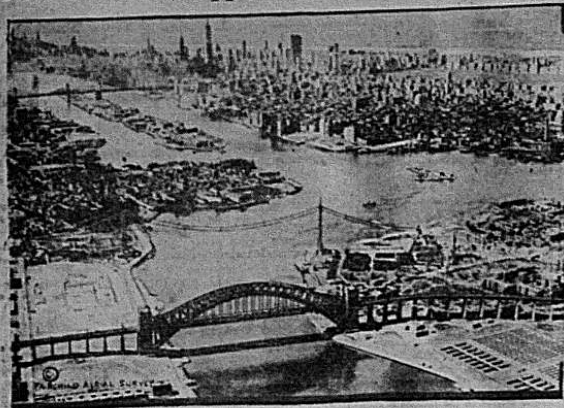
This new aerial view of New York shows the Hell Gate bridge in the foreground, linking Ward's Island, on the right, with Astoria across the East River. In the rear of the Hell Gate bridge are seen the cables for the new Triboro bridge. Farther down the river are Welfare Island and the Queensborough bridge.
