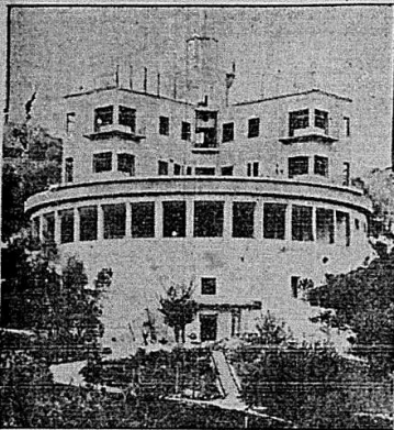
A house, the living rooms of which, as a unit, rotate on circular tracks facing the sun, making the complete turn within the arc of a circle, in 9 hours and 50 minutes. The motive power comes from a 3 horse power engine which operates in the center of the house. The house shown is situated on a hillside in Italy.
