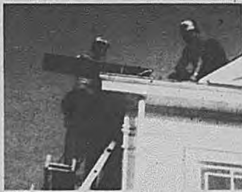
On one of the last warm days recently, working men of the Town of Oyster Bay Community Development Project at the Old Hicksville Courthouse on Heitz Place were bracing the main floor beams with a steel girder and relining the roof gutters. Jesse Stacy, left, and Mike Ahern of Unicom Ltd. are shown correcting roof leaks with new gutter inserts of copper.
