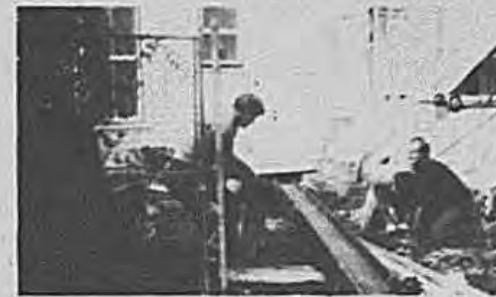
Steel workers position the girder, which was placed in the foundation walls of the Old Hicksville Courthouse recently.
