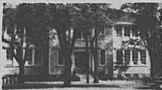
Nicholai Street School as it appeared shortly before it was demolished.
