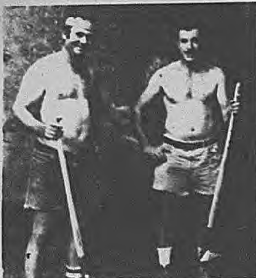
They hardly make this kind of men anymore! Mario Spilotros and Freddie Reecine who hand excavated the basement and existing foundation of the Old Hicksville Courthouse, removing old concrete and two feet of sand and gravel through a single window eight feet high. (Photos by Ed Bady)
