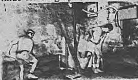
Hand excavating under the 1985 original cement foundation of the Old Hicksville Courthouse at Heitz Place was a big job for workmen Mario Spilotros and Freddie Reecine recently. The "human digging machines" were preparing the way for forms and fresh concrete to underpin the existing foundation which was poured directly onto sand.
