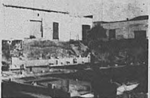
Construction of Trinity Lutheran Church's expanded facilities continues as we plan extended ministries for our members and the entire community. The new addition will bring special benefits to the youth, the elderly, and the handicapped. Trinity, located at 40 West Nicholas Street, Hicksville, cordially invites you to join us for worship on Saturday at 7:30 p.m., or on Sunday at 8:15, 9:45 or 11:15 a.m. We're here to serve! If you would like information, or we can help in some way, please call. Our telephone number is 931-2225.
