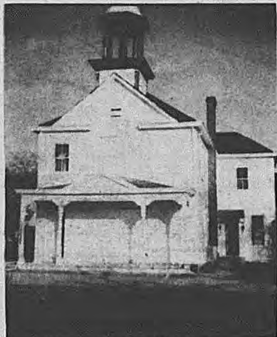
Passersby this week were treated to a bit of the traditional Maine white building vision at Hicksville's historic Heitz Place Courthouse. The home of the Gregory Museum, the 1895 building has had increased paint peeling due to leaking roof gutters. Museum volunteers used possibly the last warm spell to seal the building with white primer paint before the cold, rain sets in. The roof gutters problem is part of a Federal Community Development Project which is having bit-letting problems.
