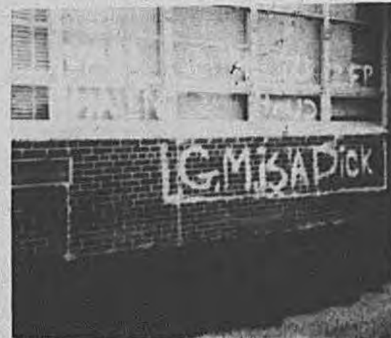
Back of Fork Lane facing Division Ave.
