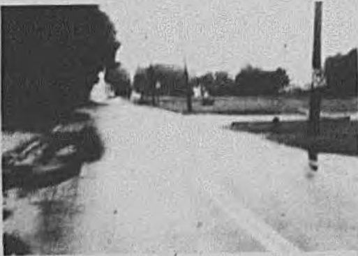
LILCO's nightmare in the wake of Gloria's passage is just beginning in this photo of electric powerline poles tilting noticeably on New South Road, facing south. Many poles will require straightening and guying, cables rehangng in weeks ahead.
