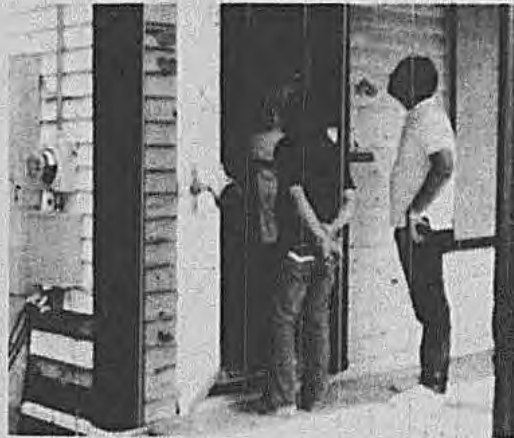
Some of the first visitors to the reopened Hicksville Gregory Museum on Sunday, July 21, inspect the front hall fire damage before touring the museum exhibits which were preserved virtually intact.
