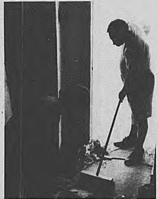
Clean-up efforts continue at the Hicksville Gregory Museum. Here, carpenter Mike Lipman and Hugh Conover, Museum Trustee (in the front doorway) remove debris resulting from a fire which threatened the Museum on June 1, following a power 'black out' in the Heitz Place neighborhood.
