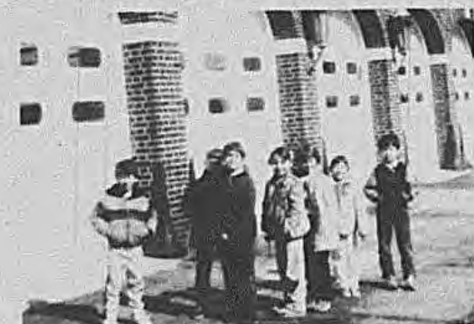
The engines were warm inside their Fire House when a few youngsters, sight-seeing Hicksville on a Fork Lane bus tour, braved cold weather to have their pictures taken by the impressive Hicksville Fire Department Building which was erected in 1932.
