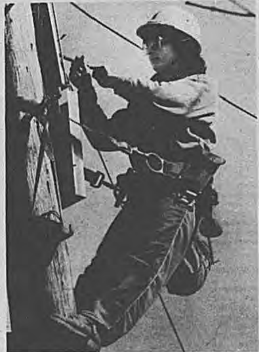
Jeanne Boccarossa of Hicksville, an installation technician with the New York Telephone Company, places a drop-wire that will deliver new telephone service to a customer. Boccarossa is among more than 200 women who hold non-traditional jobs in Nassau and Suffolk counties.
