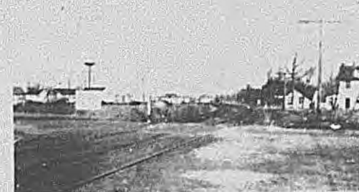
Hicksville East across Bay Ave.
