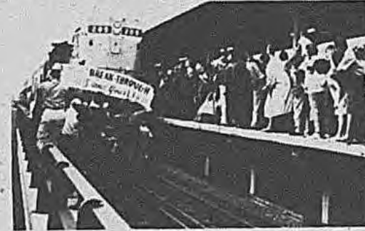
The first locomotive and cars coming in to the newly elevated Hicksville Railroad Station in 1964.
