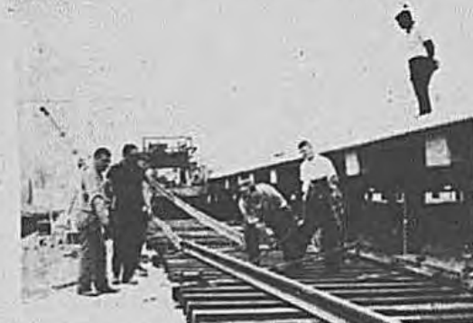
This fine photo of track laying operations at the newly elevated Hicksville railroad station in 1963 is just one of Edward Bady's pictures on display this month at the Hicksville Public Library.
