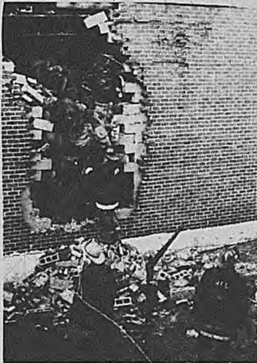
Brick wall was blown away in explosion. (HFD Photo Unit photo)
