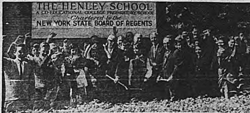
SCHOOL FACILITIES: Private, non-profit, college preparatory schools on Long Island, such as the ten-year-old Henley School at Jamaica Estates, are helping to meet the increasing demand for modern school facilities. Shown breaking ground at Palo Alto Street, in Holliswood for one of the most modern schools in the nation, to be opened next September, are directors, teachers and some of the students of Henley. To ease school shortages, three public schools and one high school, at a cost of more than $10 million, were built in Queens County last year. Plans for the future call for five more elementary schools, two junior high schools and one senior high school for Queens. Private schools like Henley, draw their student bodies mostly from Queens, Nassau and Suffolk Counties. (Graphic News Photo.)
