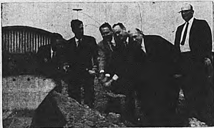
DIG THEY MUST -- Volkswagen officials break ground for the new Walters-Donaldson, Inc., authorized VW sales, service and parts facility which will be erected in Plainview at the intersection of Oyster Bay and Woodbury Roads early next year. Front left to right are Richard Skog, the agency's service manager; R. W. Josenhanns, director of sales and marketing for World-Wide Automobiles Corp., VW distributors in N.Y., N. J., and Conn.; William Strauss, the dealership's sales manager; co-owners Philip J. Walters and Jack W. Donaldson; and Mr. Walter's father, Fred Walters. Dealership will be one of Volkswagen's largest in Long Island. The firm is presently located at 277 Old Country Road in Hicksville.
