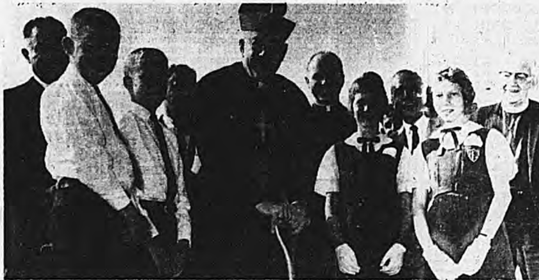
THE MOST REV. WALTER P. KELLENBERG, D.D., Bishop of the Diocese of Rockville Centre, this week broke ground for the last of four new high schools planned for construction in the largest single undertaking in the history of the diocese.
