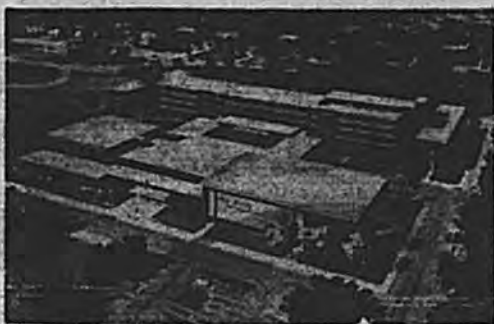
ARTIST'S VIEW of Holy Trinity Catholic High School to be built in Hicksville. School will have enrollment of 2400 students.
