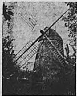
When you reach East Hampton you turn left just before you reach this historic landmark, an old windmill built in 1805. The hand-hewn wooden gears that turned the old millstones are well preserved. The windmill is open to the public.
