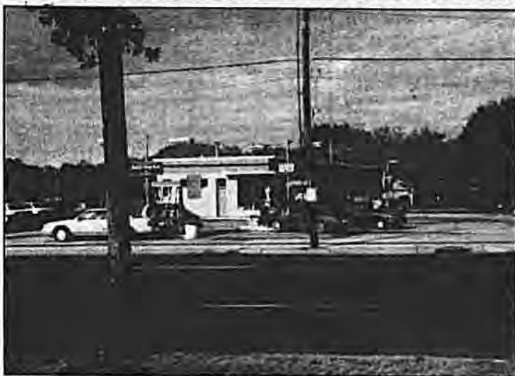
SHELL IS LOOKING to tear down the existing gas station and rebuild it adding a food mart. The Town of Oyster Bay has taken the petition under consideration.
