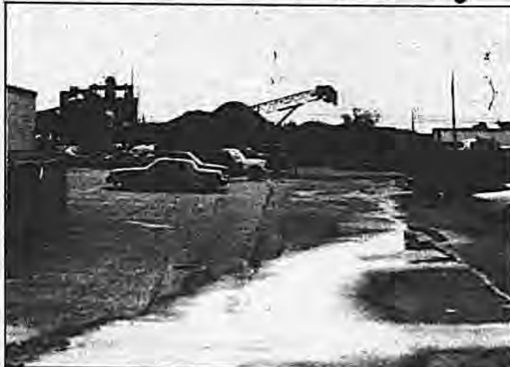
IN THE DISTANCE stands the Twin County Recycling Plant. A recent court decision said that the plant was not in violation of any laws and can continue to stay open for business. (Photo By Victor Caputo)
