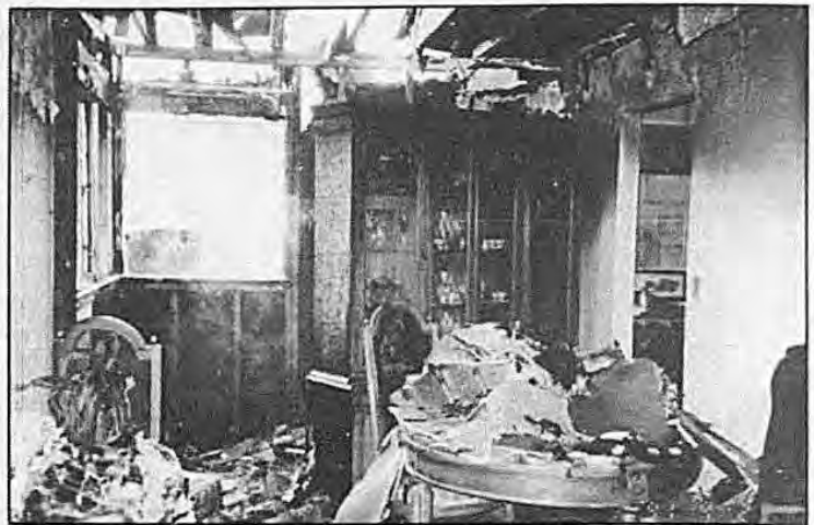
INSIDE OF the home on Fox Place which was partially destroyed by fire.
