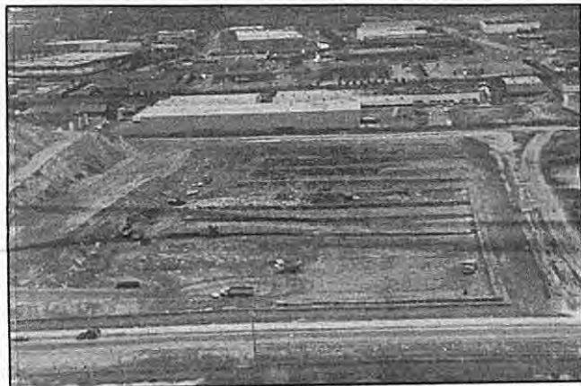
MANAGING THE WASTE STREAM: Throughout parts of North Hempstead, pungent odors from the Port Washington landfill—shown in this aerial view—irritated hundreds of residents nightly. From recycling to incineration, Nassau County faced difficult choices in dealing with its waste materials during 1990.
