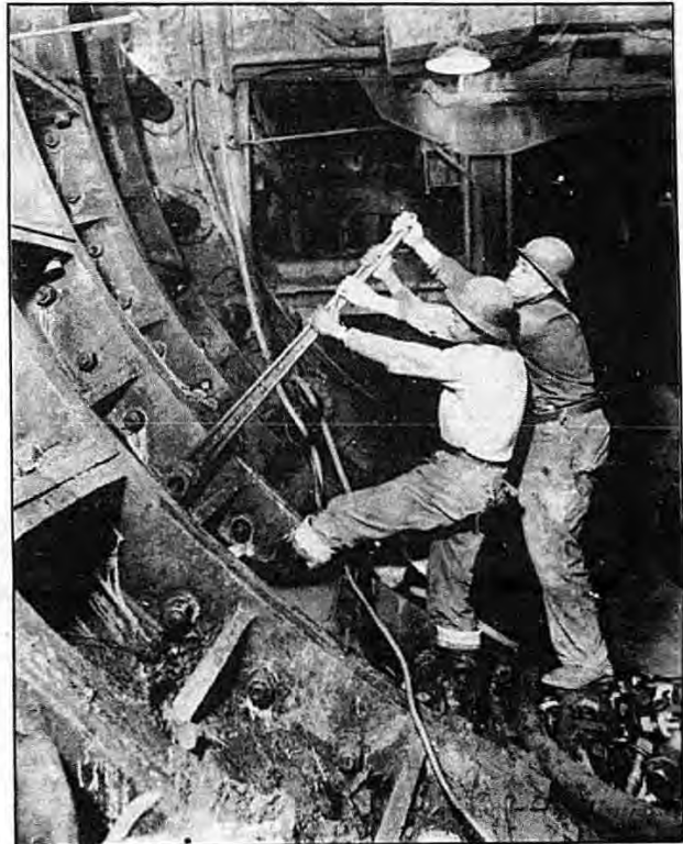
SCARED OF TUNNELS? IMAGINE how the 'sandhogs' who built them felt. These two gentlemen are tightening a tunnel bolt with a five foot ratchet wrench, on February 26, 1939, during construction of the Queens Midtown Tunnel.
