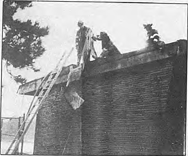
Firemen "peel" the roof of the building to find the fire trapped in pockets.
