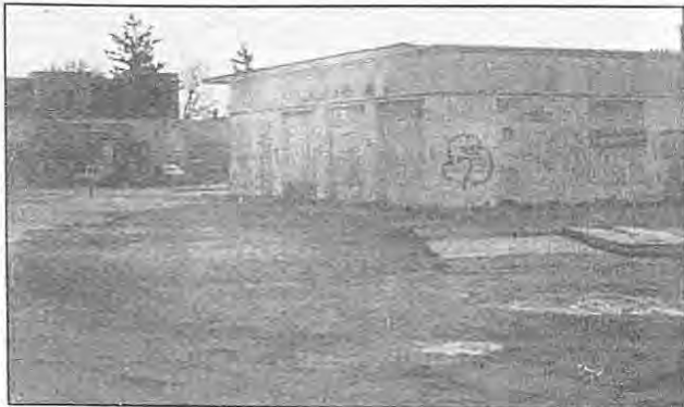
This gas station on North Broadway at James Street, near the mall, has been abandoned for years. In Nov. 1989 the owner of the gas station requested a permit from the Oyster Bay Town Board to convert the building into a self-serve station and convenience store. A town spokesperson said Friday that the town board is continuing to review the application which includes an environmental review. This is a typical review process for any application before the town board decides whether to approve or disapprove the permit.
