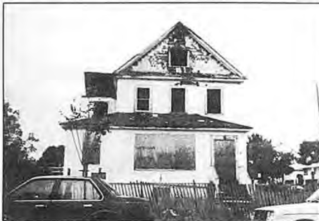
Vacant house on corner of West John and Strong Streets. A local developer plans to demolish this house and replace it with an office building. The house was damaged by a fire a few months ago.
