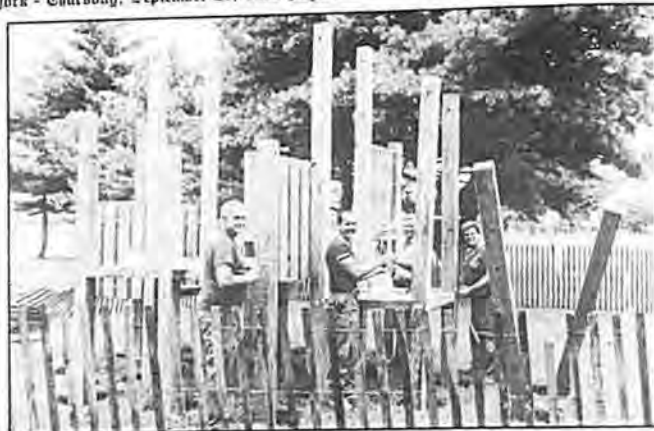
Town of Oyster Bay workers construct a Jungle Gym as part of a new playground that is being installed at the Abe Levitt field on Stewart Avenue near Dutch Lane School. The Jungle Gym comes complete with swings, slides, sliding poles, ramps, and overhead ladders.
