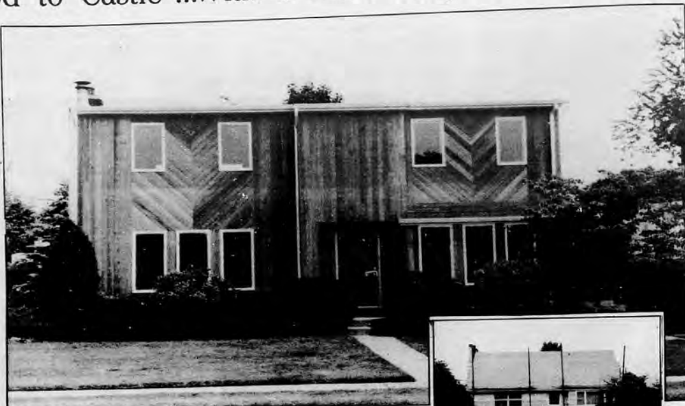
NEW HYDE PARK Cape goes modern. Larsen added a second story, utilized vertical and herringbone cedar siding and long, rectangular low E windows to create a contemporary home with a spacious feel. The vertical lines give added height and architectural balance.
