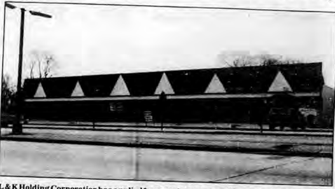
L & K Holding Corporation has applied for a special use permit to use this building, across from St. Ignatius Church, for retail purposes.
