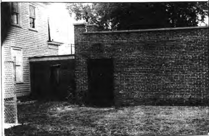
THIS JAIL HOUSE is connected to the back of the old Hicksville Court House (now the Gregory Museum). The jail was built in 1915 and was used until 1935 when the last inmate took his life.
