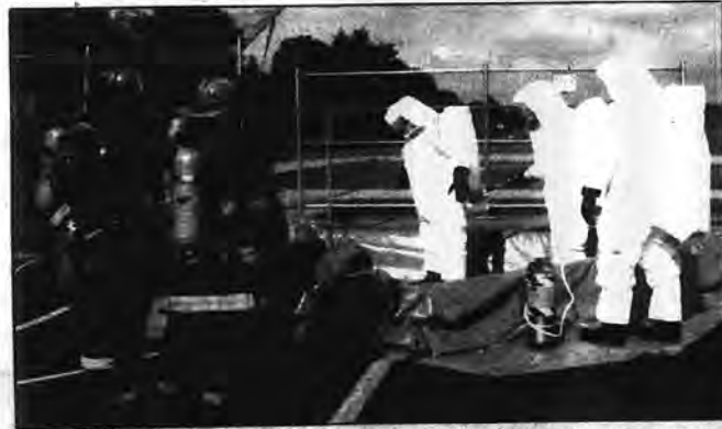
HAZ MAT TEAM members at a decontamination scrub-down after they removed chemicals from a loading dock at the Hicksville School's Administration Building.
