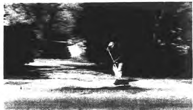
BUT ON THE OTHER side of Woodbury Road is this "eye cure;" a workman sweeping loose sand and gravel.
