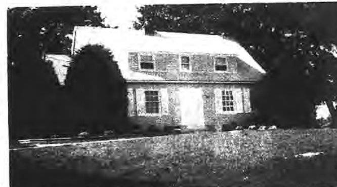
DEMONSTRATING THAT responsible business leadership can contribute to the appearance of Hicksville are the modernized cottages on South Broadway, which were recently converted into offices. These structures were formerly part of the Hartmeier homestead, one of Hicksville's farming families.
