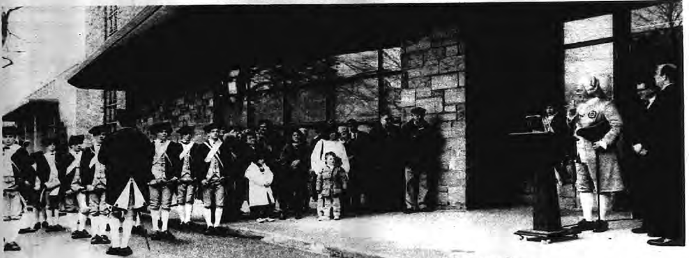
WILLIAMSBURG FIFE AND DRUM CORPS IN MANHASSET: B. Altman and Company department store, located on Northern Boulevard in Manhasset, was the site of a performance by the renowned Williamsburgh Fife and Drum Corps on Friday afternoon, Nov.
