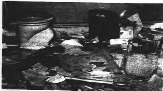
GLASS AND DEBRIS in vandalized, abandoned courthouse.
