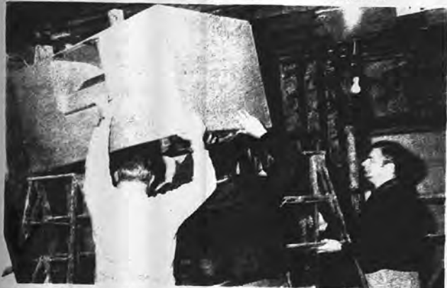
IRWIN BOTTO , of Botto Mechanical Corp., supervises sheet metal workers, Union 55, putting in air conditioning. Irwin served for many years as Museum Trustee and Generous Benefactor.
