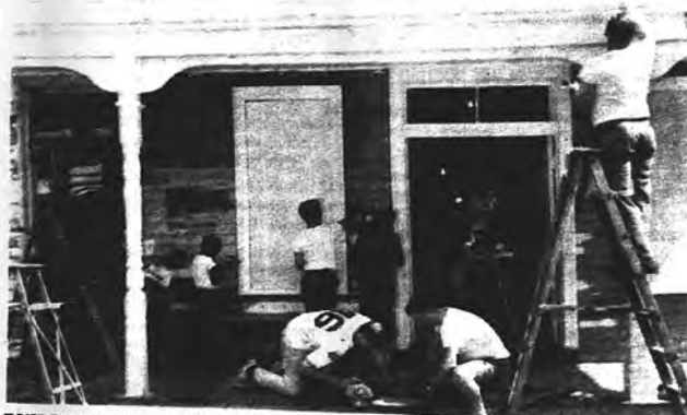
BUILDING CHAIRMAN Hugh Conover and Volunteer Frank Larkin work on courthouse porch. Co-chairman John Strong is on ladder.
