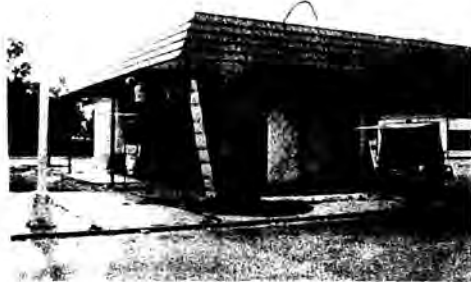
Shows here is the Renovation being done to the main entrance of the Galileo Lodge on Levittown Parkway Hicksville.
