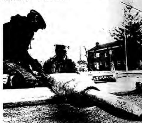
A "Russian Missile" is being readied to carve out a tunnel for an underground electric line beneath Wellwood Avenue in Lindenhurst. Pat Cannon, left, and Warren Brown of the Long Island Lighting Company's Underground Lines Department are setting the controls.
